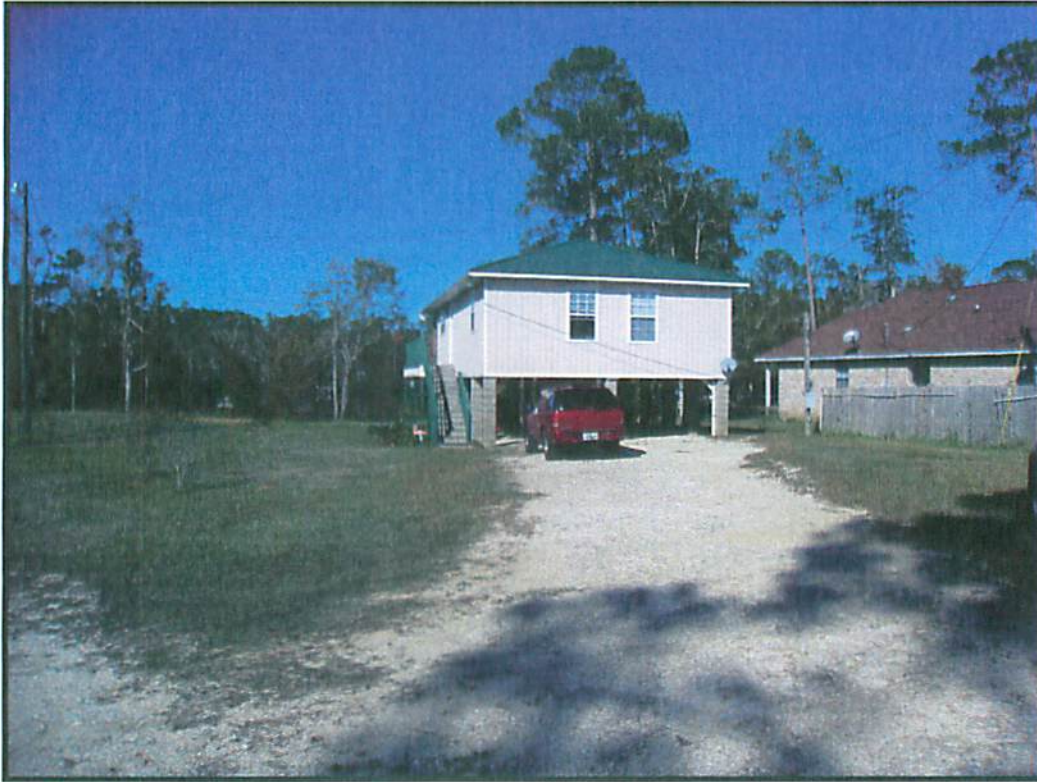
NORTHERLY VIEW TO PROPERTY - TAKEN FROM SERVICE ROAD
