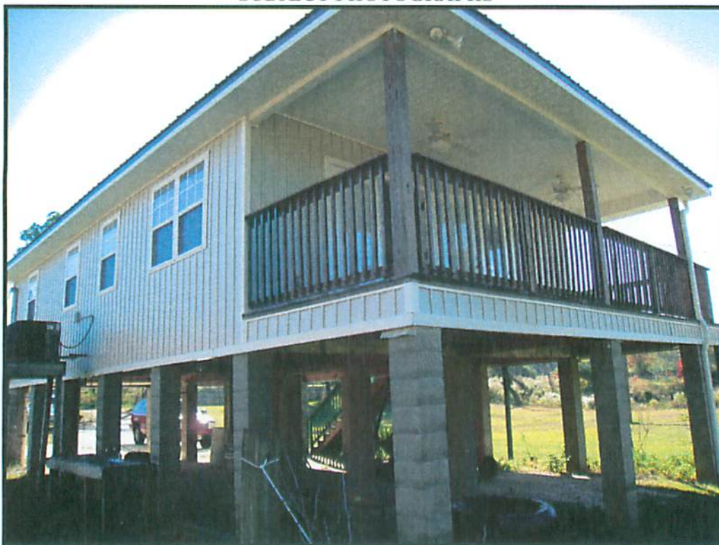
SOUTHWESTERLY VIEW TO REAR/SIDE OF RESIDENCE
