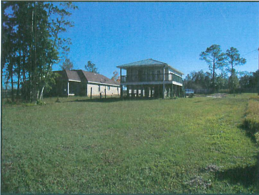
VIEW TO PROPERTY FROM NORTHWEST CORNER
