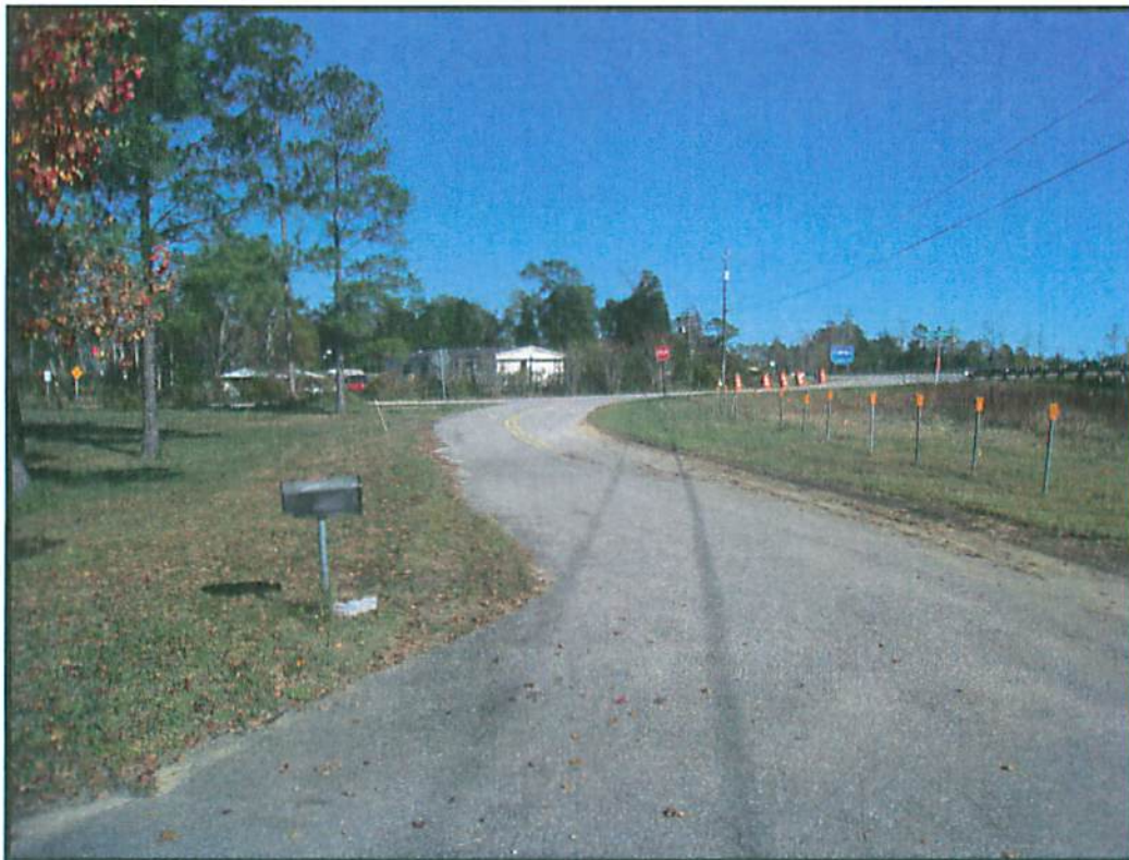
EASTERLY VIEW ALONG SERVICE ROAD FOR MOBILE HIGHWAY
